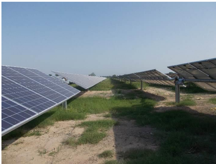
Figure –2: Solar PV plant with HSAT installation
