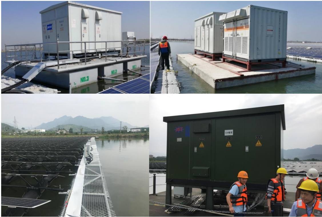
Figure 3: Floating platforms for central inverters, string inverters and transformers
