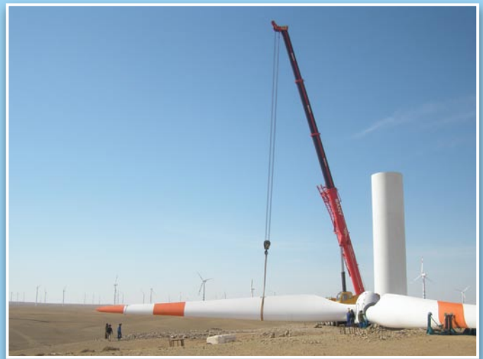
WTG installation at Bailingmiao, Inner Mongolia.
