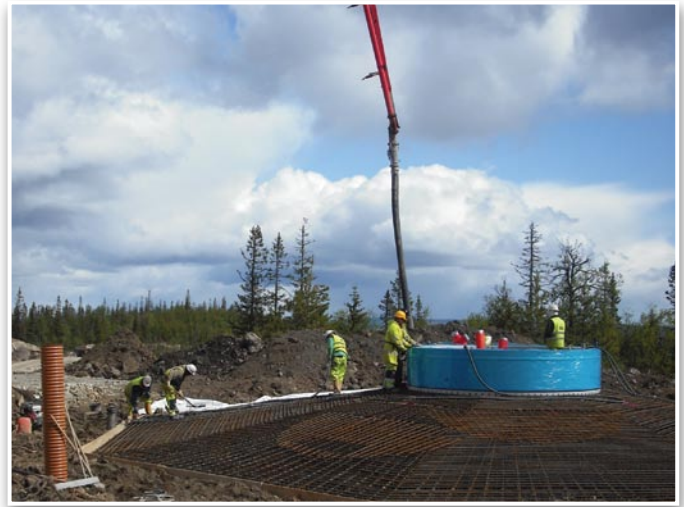
Foundations being poured at Havnäs wind farm, Sweden
